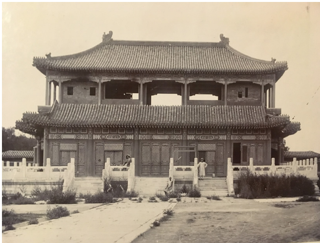
Fig. 10: Hall of Imperial Splendour ca. 1901, the upper floor without exterior walls Photograph, private collection.
